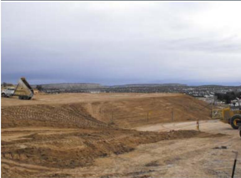
All waste material, except asbestos, was brought onto the mine site, contoured, and seeded. Erosion control is maintained until final site remediation in the future.
