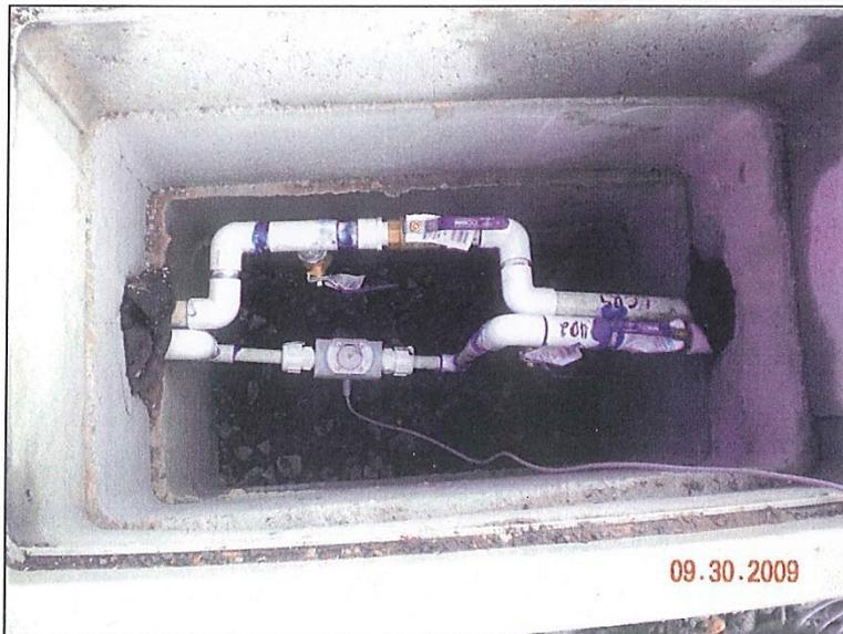
Photo 12. Looking down at new HD-2 flowmeter and LCRS monitoring ports.
