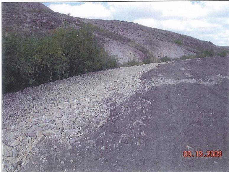
Photo 10. West drainage completed, looking north.
