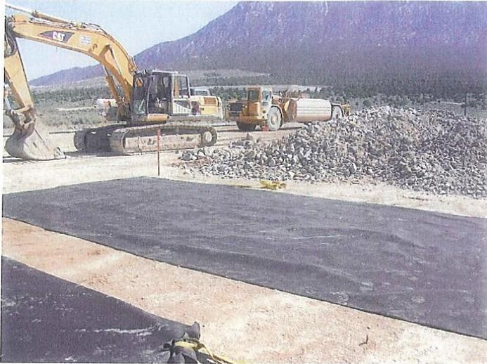
Photo 3 – Fabric Placed Over Liner Pairs
