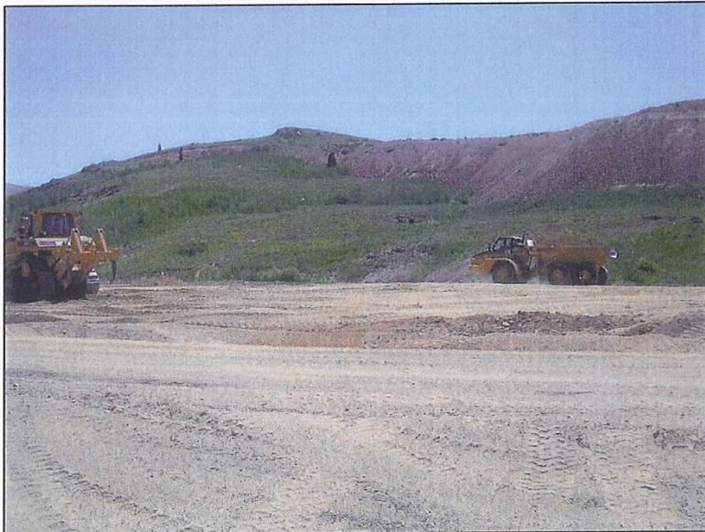
Photo 2. Hauling spent ore to middle of heap and spreading with dozer.
