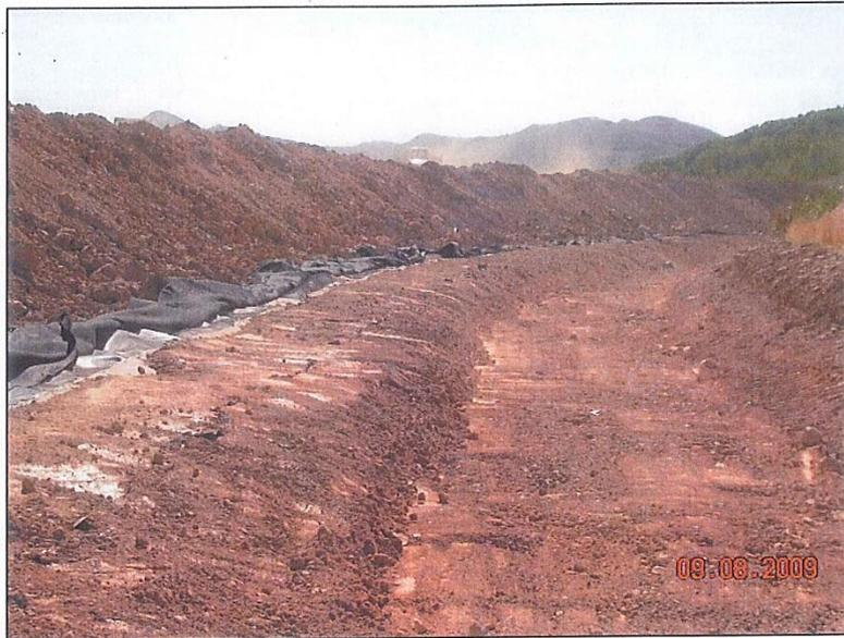
Photo 9. West drainage prior to geofabric and geocomposite placement, looking south.
