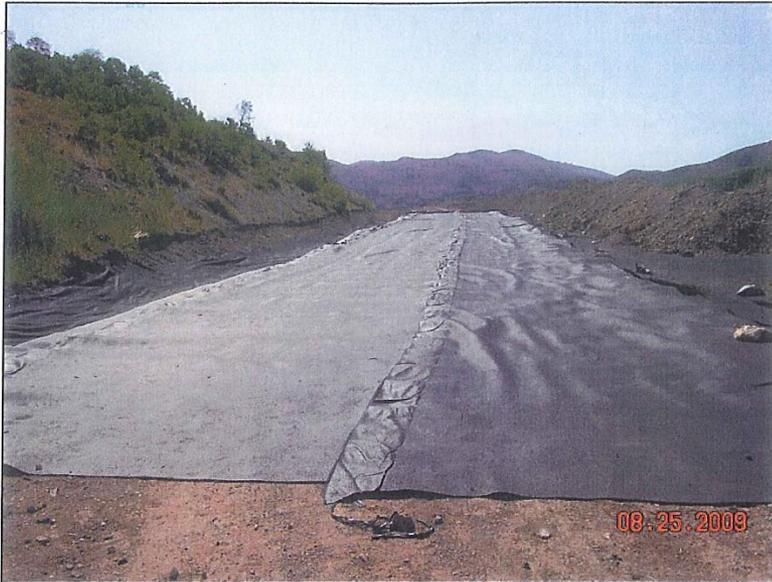
Photo 7. Geocomposite and geofabric placed along road and east drainage, looking south.
