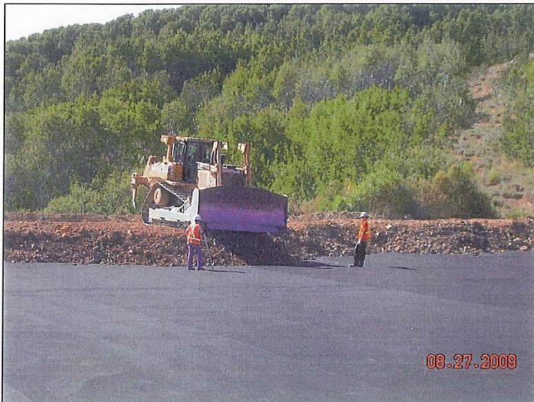
Photo 8. Spotters used during cover fill placement.
