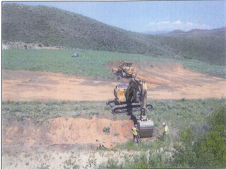
Photo 1. Exposing existing liner edge and dozer stripping topsoil.
