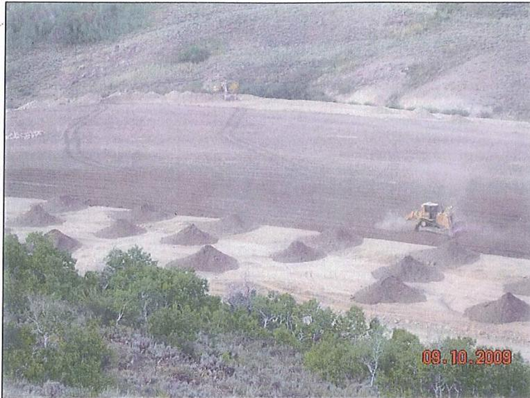
Photo 11. Topsoil being spread over the top of the cover fill..
