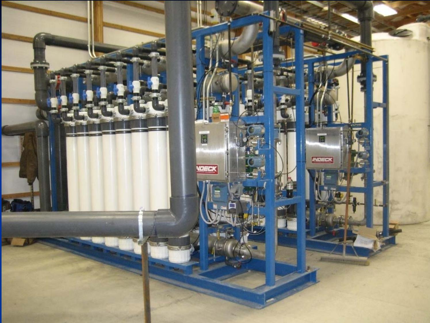
500-gpm UF system at Montanore Mine
