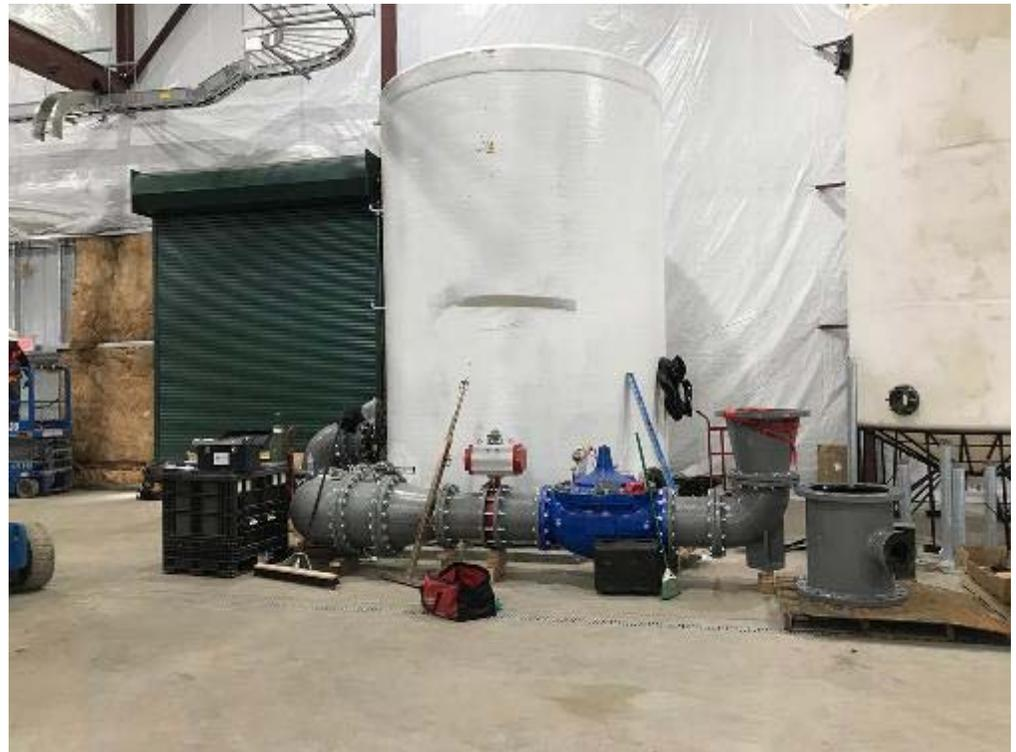
Single Stage Operation: High pH filtration. Used when aluminum is low and RO not needed. Limited to 6 MGD.
