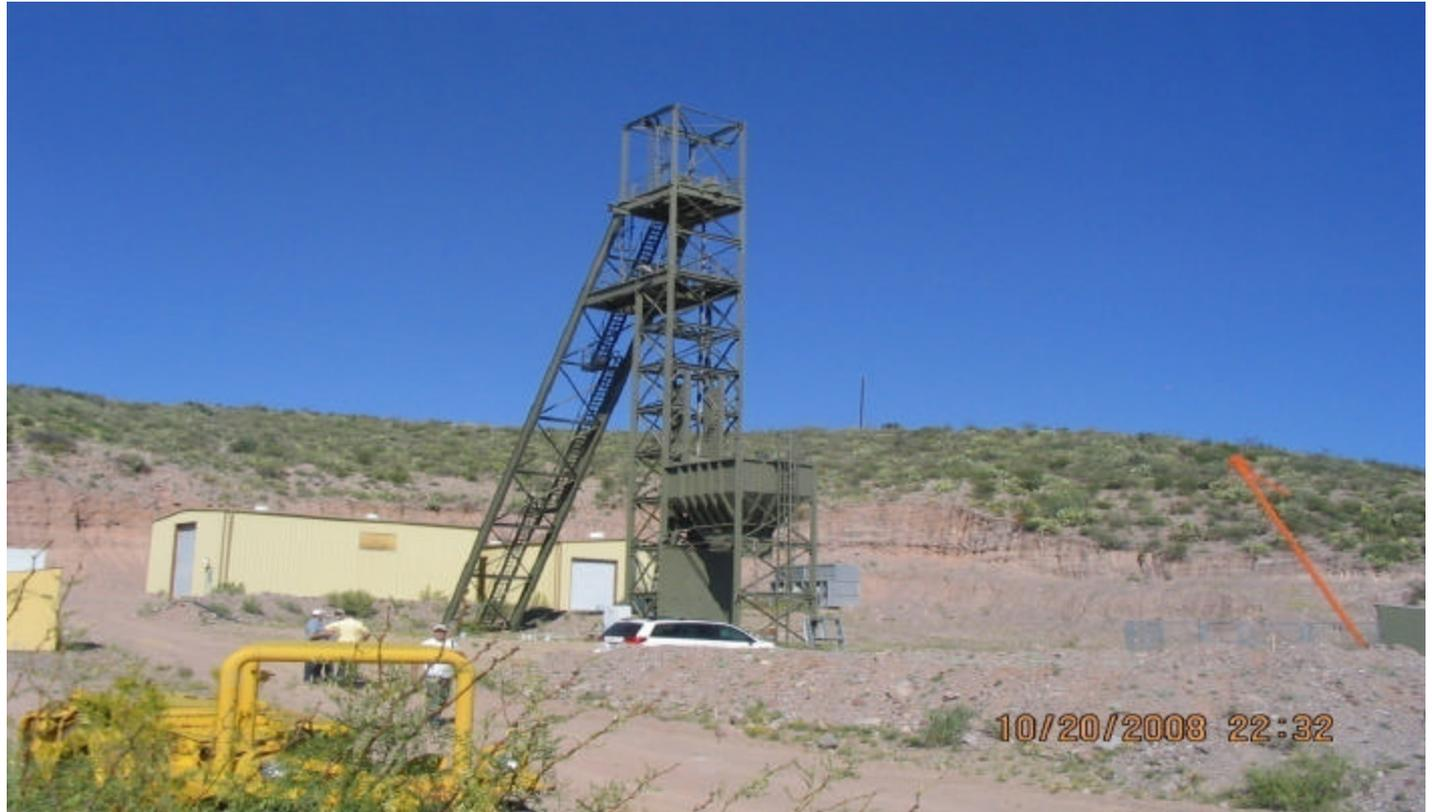
Vertical Shaft, Headframe and escape way in place
